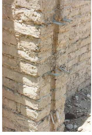
*rush matting*, lain vertically and horizontally, in the walls. The base of the vertical rushes, which is to be submerged in the foundations, features nails jutting out in every direction,
