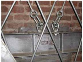
holes just existing in the masonry. The aim is to "*confine*" laterally the walls adding horizontal loads, thus connecting the various vertical layers of the masonry. As seen, the more expensive stainless steel material is used in the areas which are most exposed to the air and most closely in contact with the old masonry.
