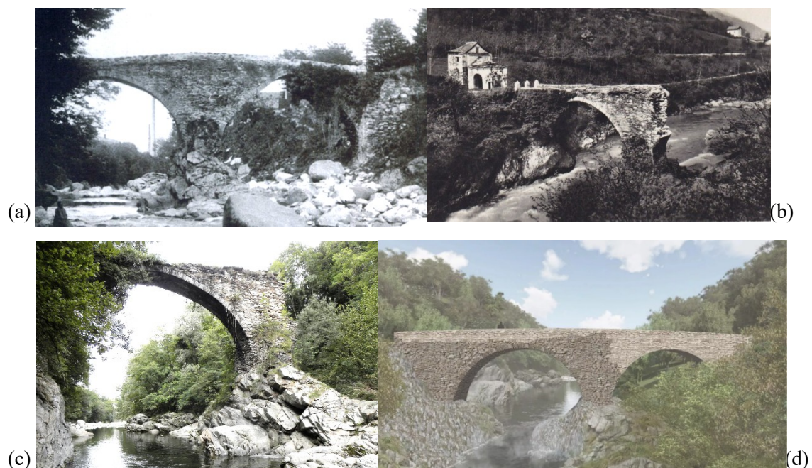
Figure 1. Life of the bridge (a) in the early 20 th century (left); (b) in 1952 after the collapse (right) of the eastern span; (c) conditions prior to the restoration works; (d) rendering of the restoration project.
